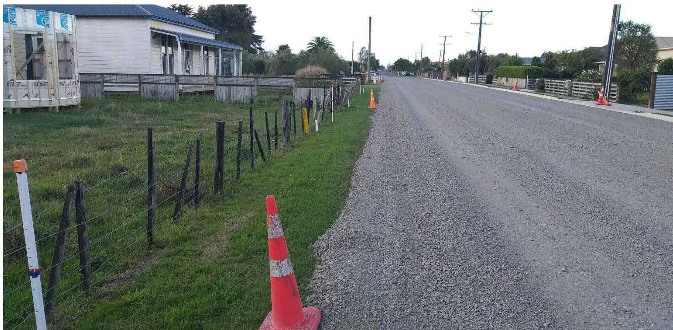
Photograph - The swale drain/table drain referred to above is evident along the current fenceline. Further south of this location it enters undulating land and is not visible.
