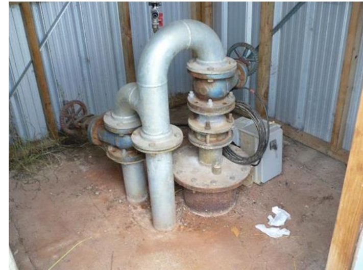
Figure 7 - Frederick Street Bore
