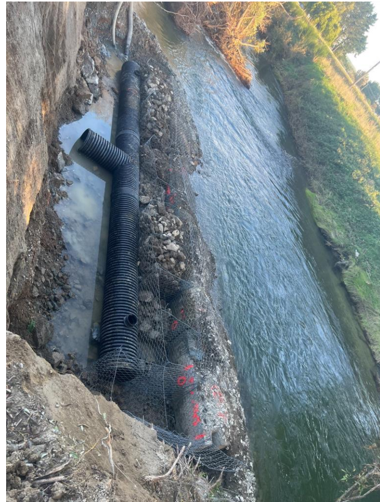
Figure 11 - Wastewater outfall structure within Mangatarere Stream
