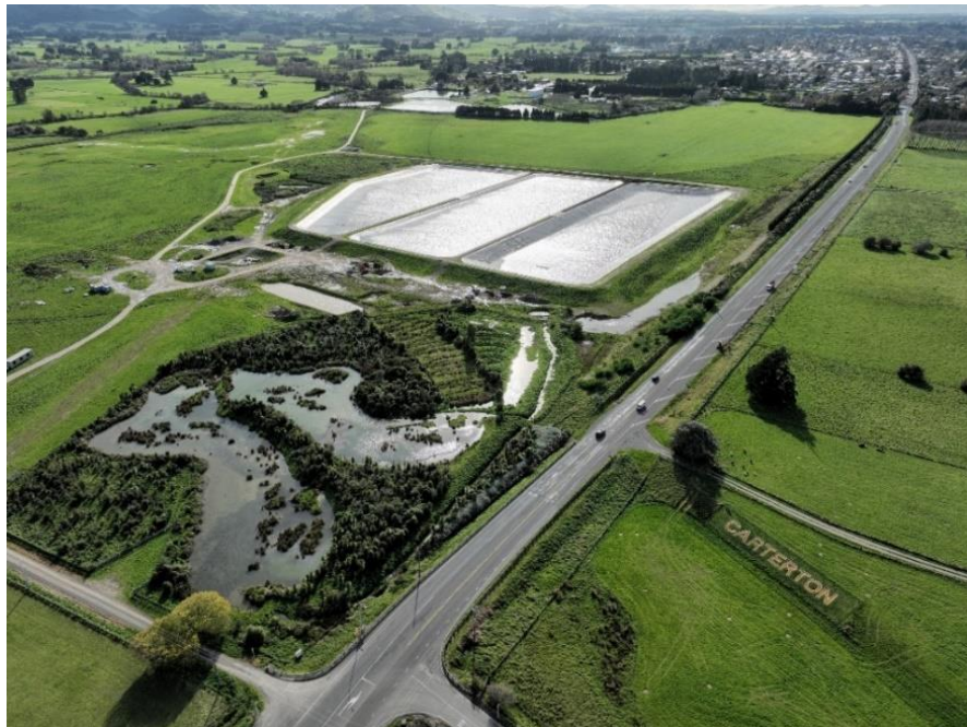
Figure 12 - Carterton's wastewater effluent storage and dispersal field
