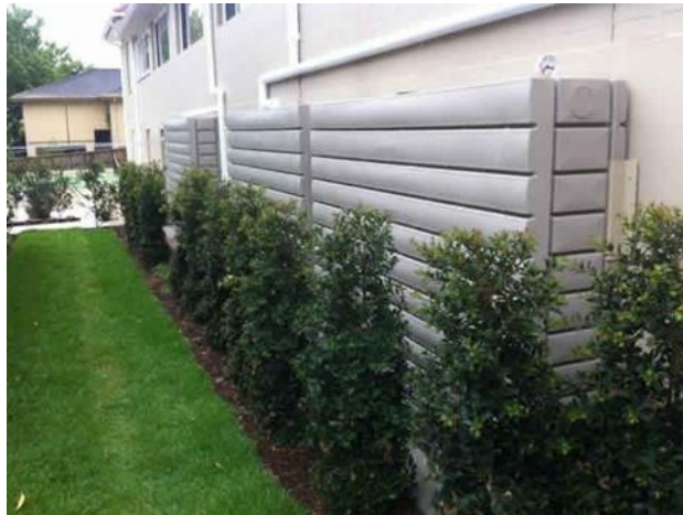
Figure 19 - An example of a modular stormwater storage cell
