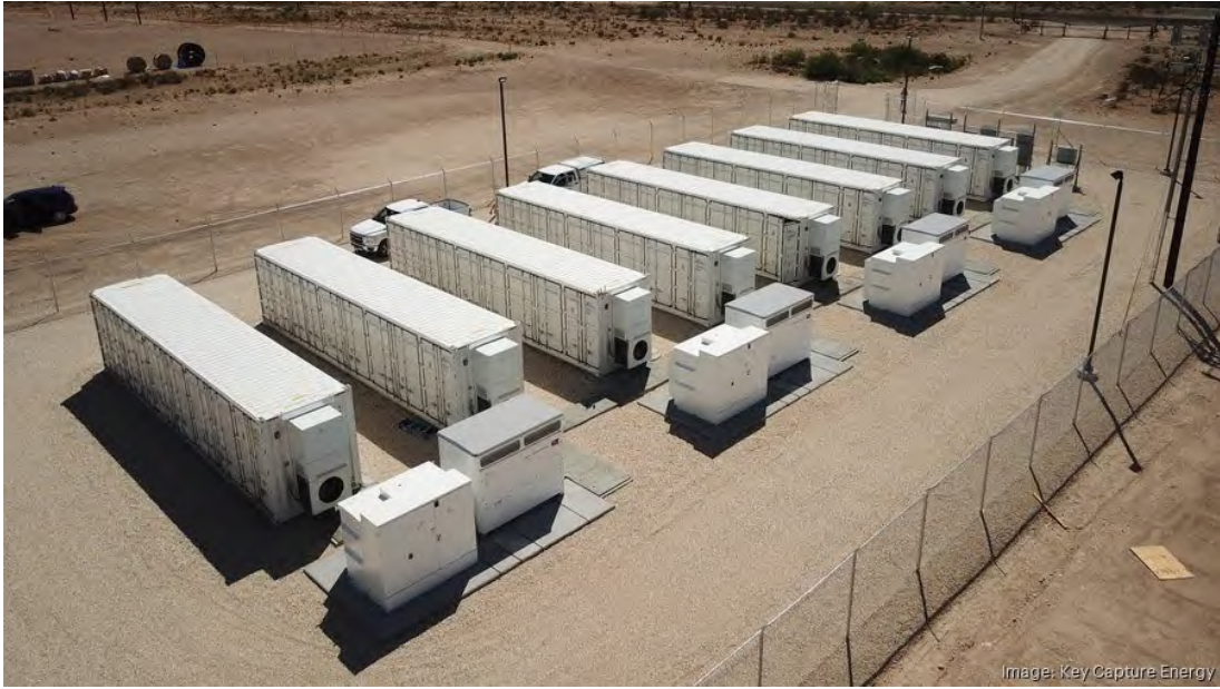
Figure 4: Example of BESS Units.
