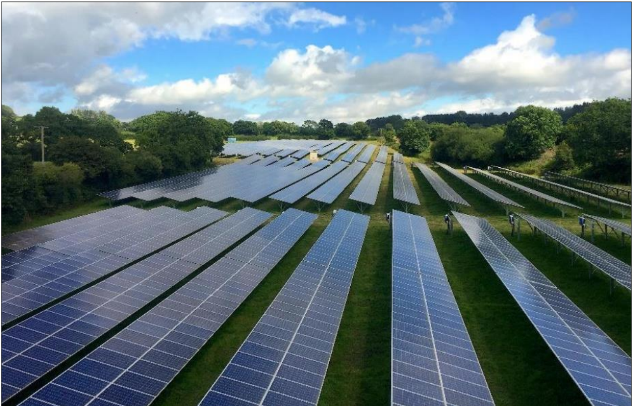
Figure 3: Example photograph of ground-mounted solar arrays
