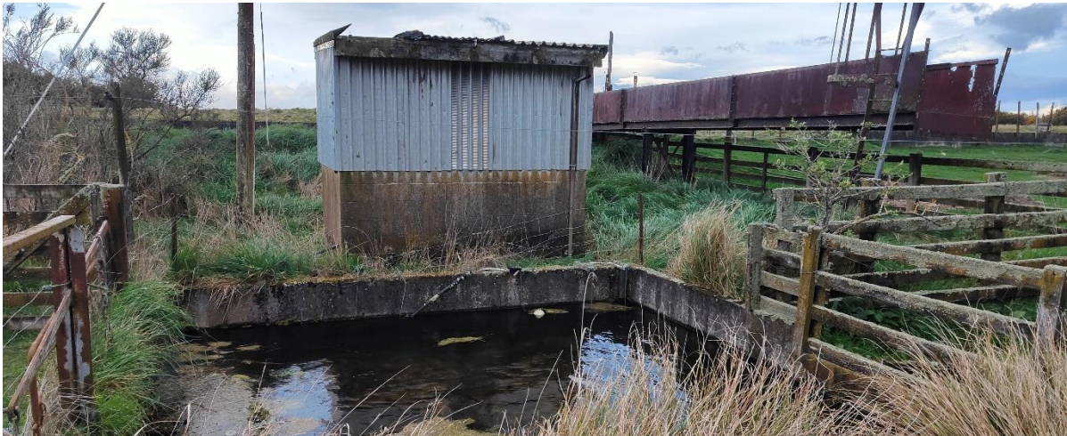
Figure 18: Historic freshwater bore and pump shed.
