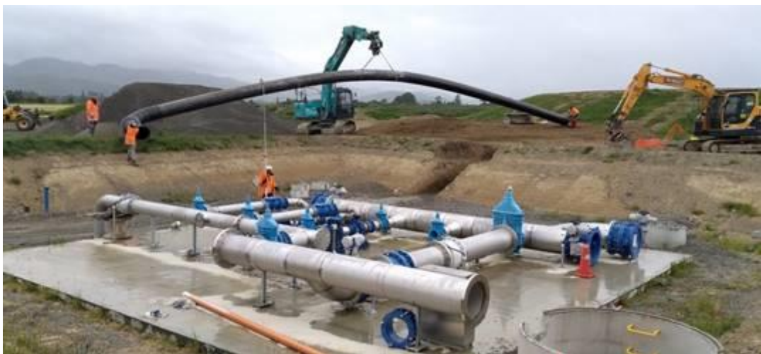
Image 7 – Reservoir outlet constructed
