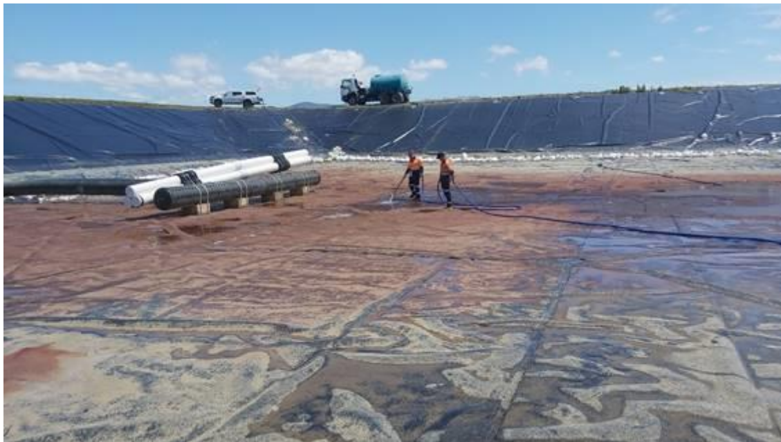
Image 8 – electrical leak detection
