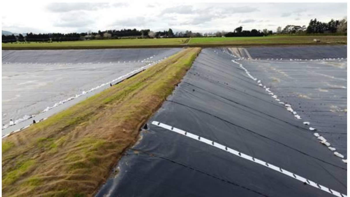
Figure 2: Topsoil and grassing of crests
