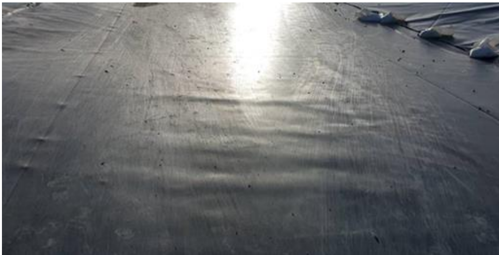
Picture 2: Scratches to the liner with what appears to be drag marks (Potentially digger bucket drag marks)
