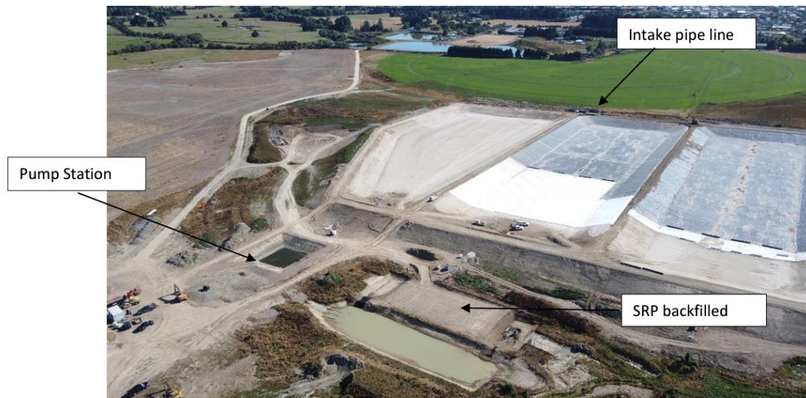
Figure 4: 12 th Feb showing pump Station intake pipe location.
