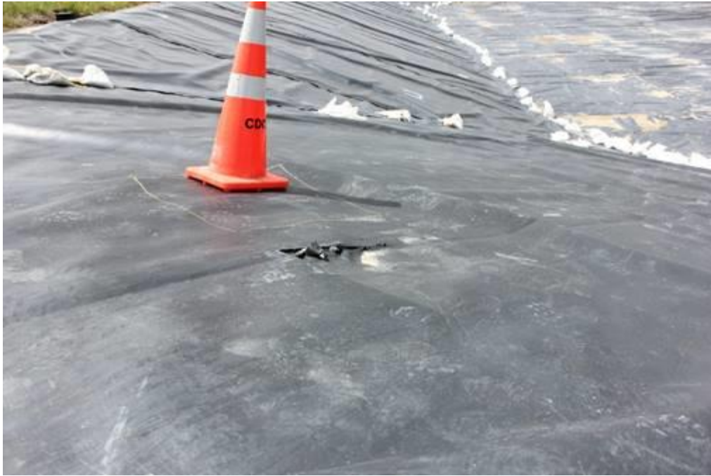
Picture 3: A tear to the liner on a corner embankment.
