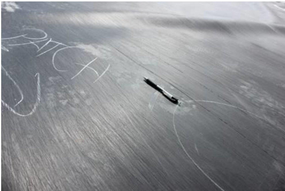
Picture 4: A closer view of scratches with a deeper longitudinal scratch apparent in the liner.
