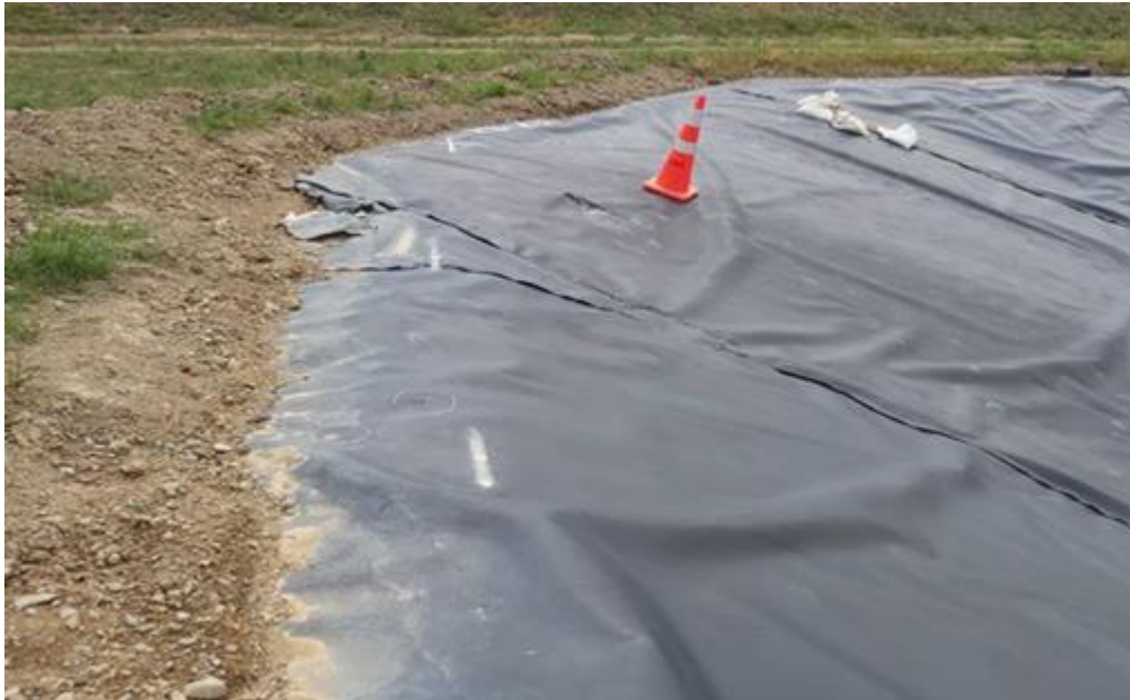
Picture 1: Liner damage at the top of the embankments on one of the reservoirs
