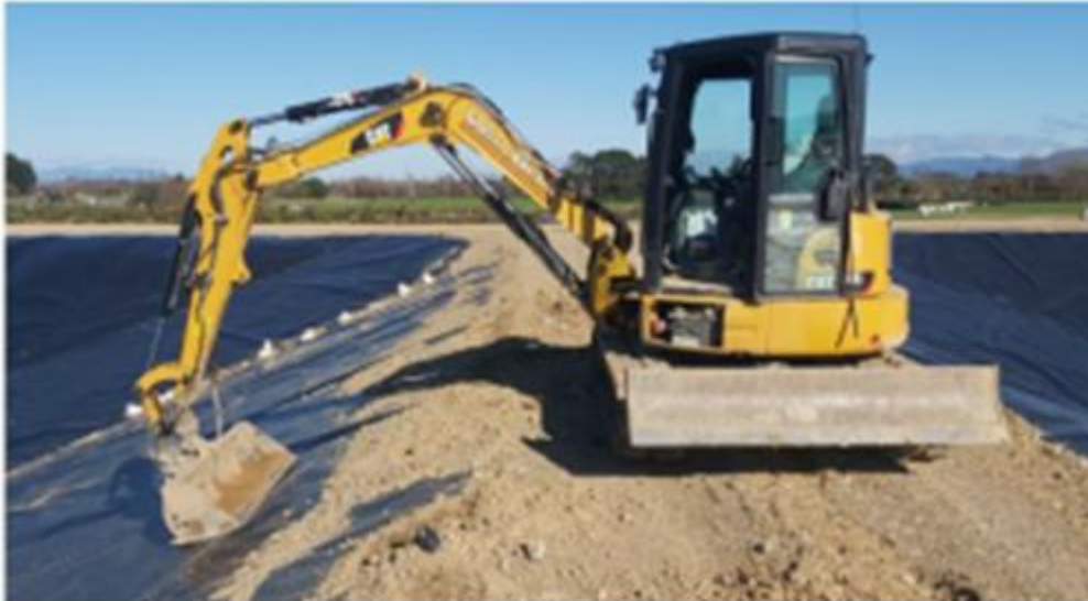
Picture 5: Excessive soil coverage at the top of the embankment and digger bucket resting on geomembrane liner.
