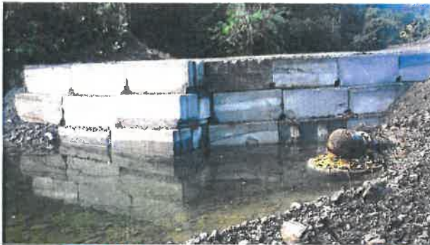
Dam head wall after new outlet pipes installed.
