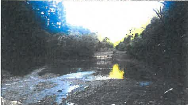
Looking down into dam, from western end.
