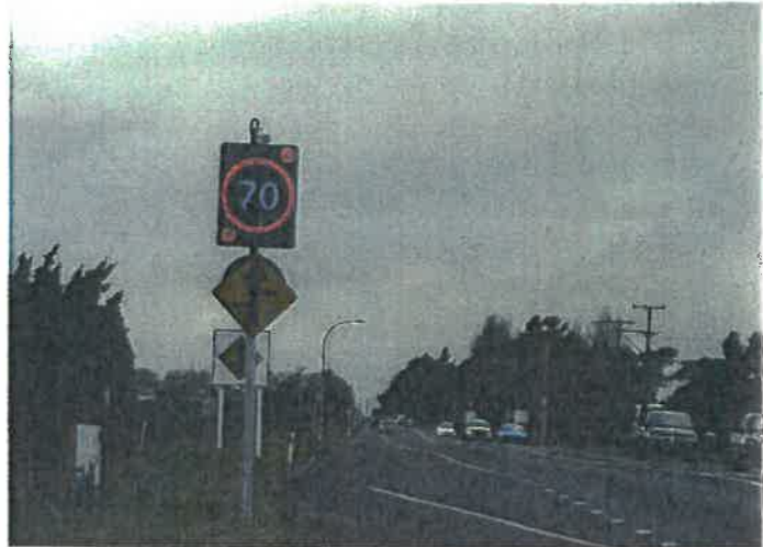
A State highway 2 variable message sign at Wiltons Road/ East Taratahi Road; the speed limit reduces to 70 km/ h when a vehicle is waiting to leave a side road.
