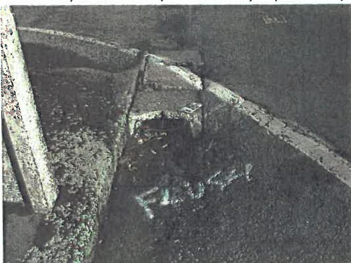
Drainage channel on High Street South at Moreton Road
