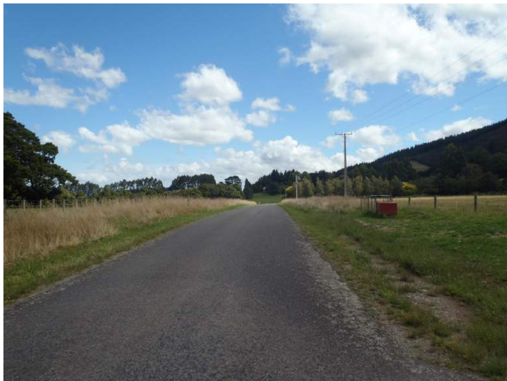
Figure 2: View of Dalefield Road looking west
