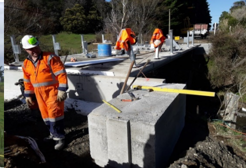
New Structure in place
